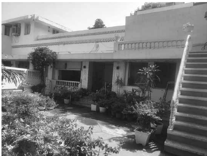
LEFT: Bhatia House and gate post. Photographs Vijay Massey 2023.
